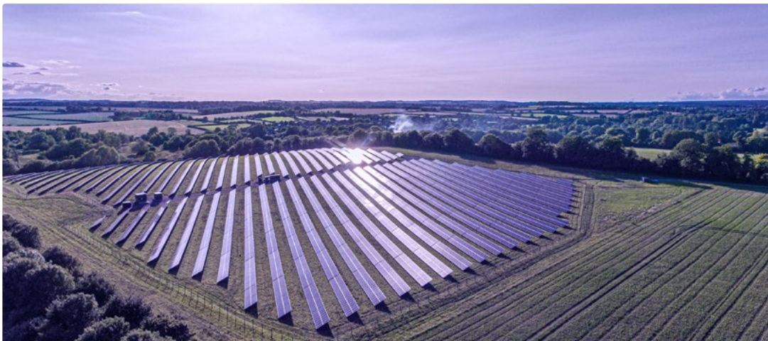
Octopus-managed solar plant in Hampshire, generating 4.5GWh/annum.
